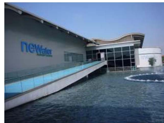
Bedok Newater visitor center
